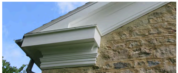
SW cornice and gutters, after restoration
