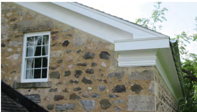
NW cornice, window and gutters, after restoration
